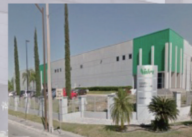
Control System Factory-KDM (Mexico)
