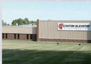
Hydraulic Elevator- CANTON (Ohio, USA)
